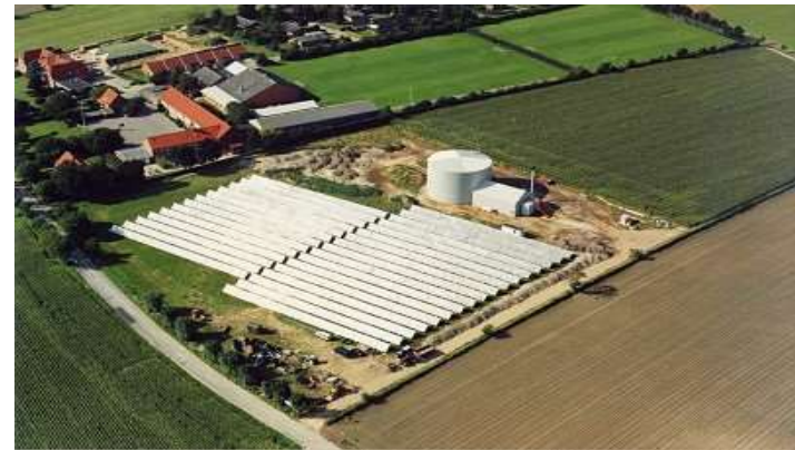
Rise 4 000 m 2 / 2,8 MW Solar fraction 45% with steel tank. Combined with wood pellet boiler
