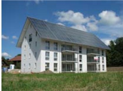
Figure 19: 100% solar heated multi-family house in Switzerland. Installed capacity 193 kW<sub>th</sub> (276 m<sup>2</sup> collector area) and a 205 m<sup>3</sup> heat storage.
