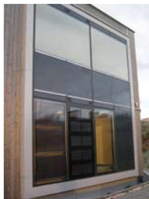
Figure 30: integral solar-active facade (right). (Source: www.smartfacade.nl)
