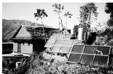
Fig. 13b: Solar water and space heating in
