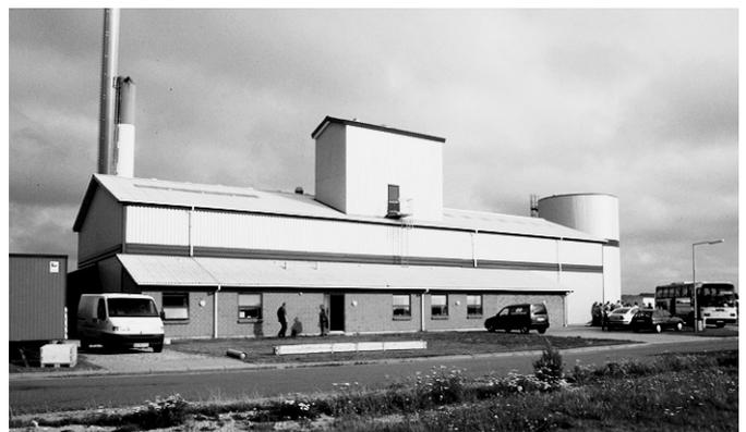
Fig. 5b: Community combined heat and power (CHP) plant, fueled by wood chips, for 300 families in Denmark
