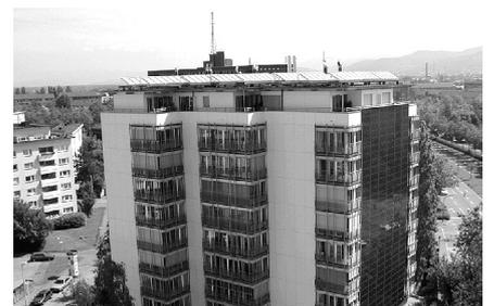
Fig. 16b: A multifamily building in Freiburg, Germany, using the roof for solar water heating, and the south wall for solar electric energy production.
