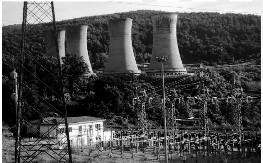
Fig. 7: Where world geothermal power production first started, Larderello, Italy. Site of the first experiment to use geothermal steam to produce electricity, on July 15, 1904, then site of the world's first geothermal power plant, 250 kW<sub>e</sub>, in 1914. Larderello, located on the hottest geothermal spot in all of Europe, today produces about 400 MW net of geothermal electric power.
